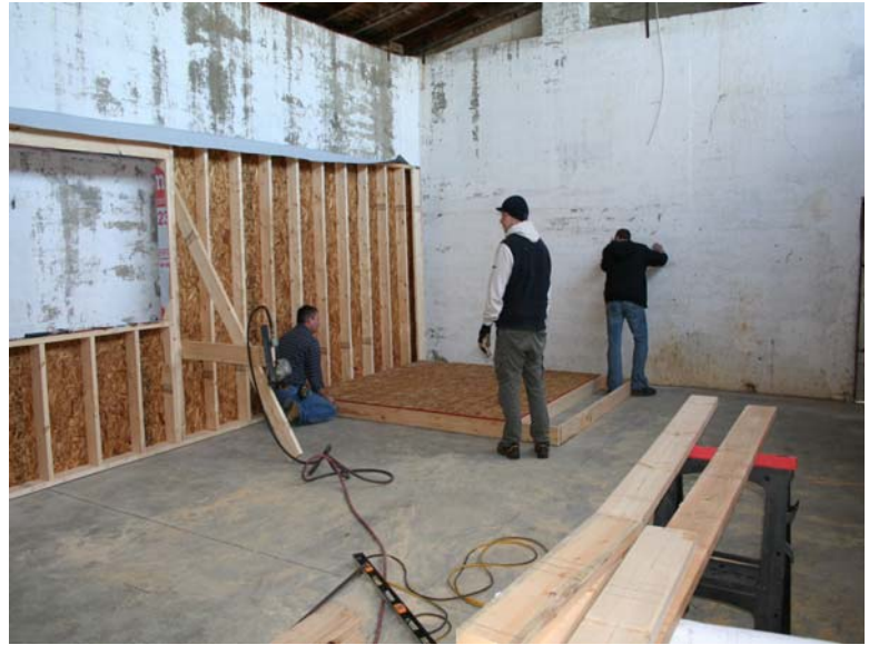
Framing of Test Facility
