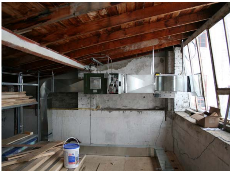
Air Handler Installation Completed
