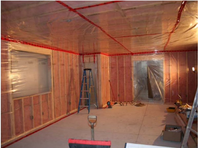
Insulation of Test Facility
