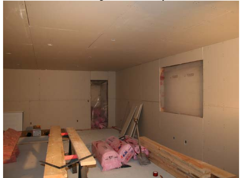
Test Facility Dry Walled
