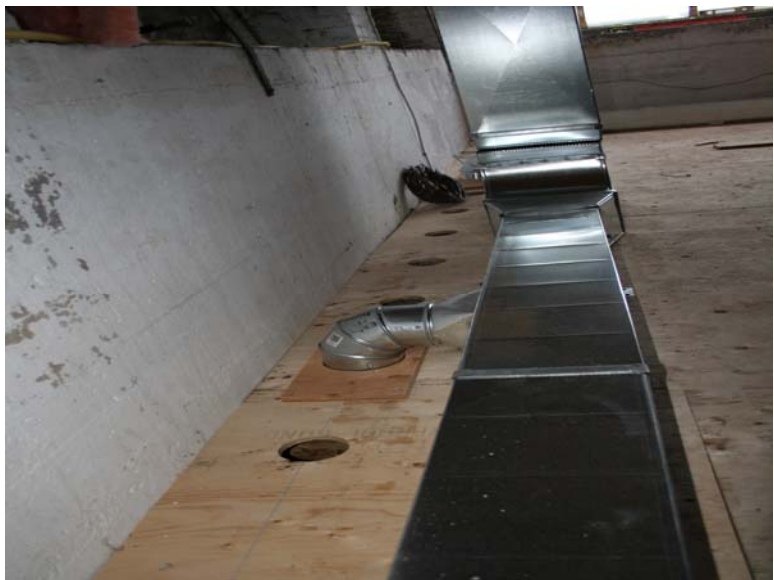
Air Gap Supply and Return Ducting
